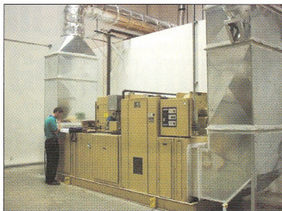
Figure 3. Example of a dehumidification system installed for a diagnostics dry room.
