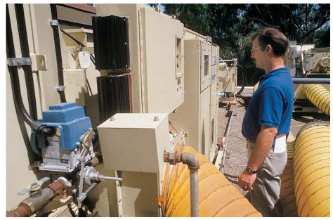
Munters' temporary humidity/temperature control system was built up from equipment hoisted on to the Museum roof with a crane. It kept an area nearly 400,000 cubic feet at 72° F and 55% RH.
