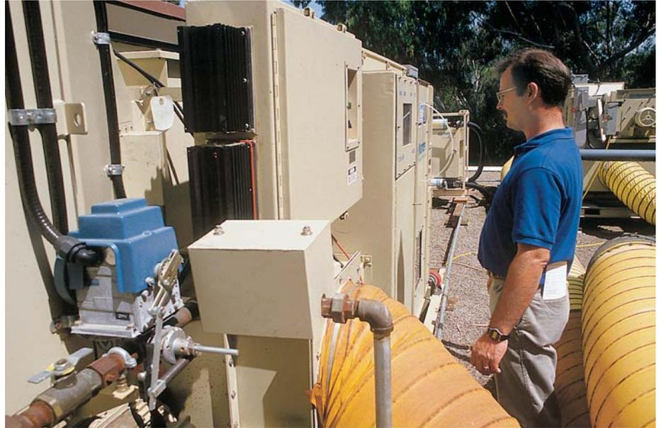
*Munters' temporary humidity/temperature control system was built up from equipment hoisted on to the Museum roof with a crane. It kept an area nearly 400,000 cubic feet at 72° F and 55% RH.*
